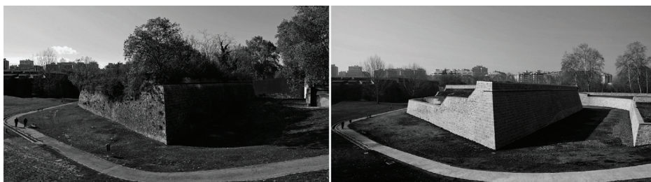
Figure 9. Santa Ana Ravelin: before and after the restoration works.
