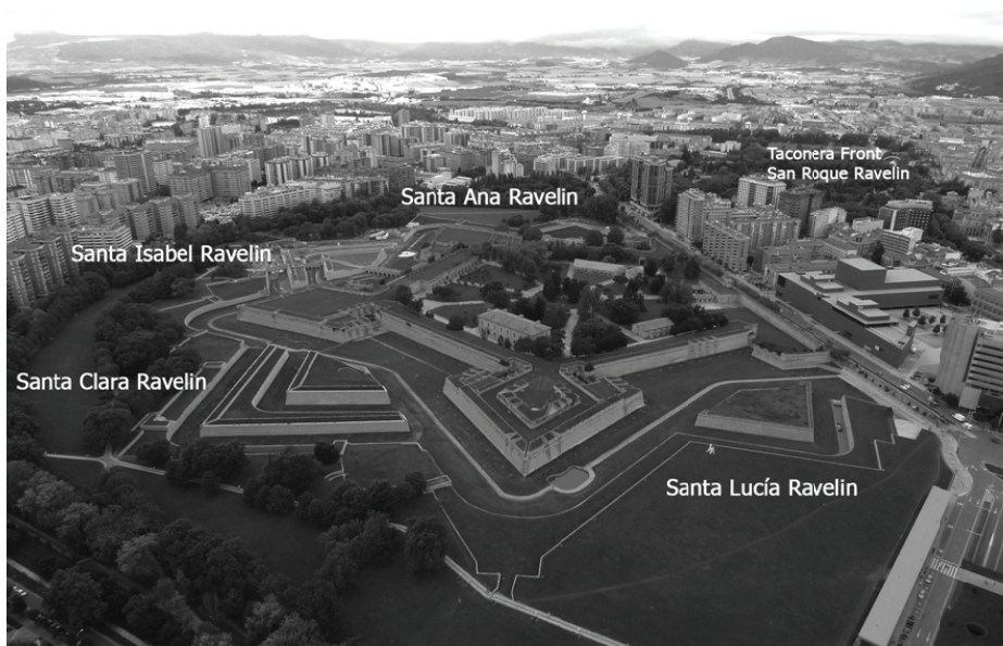
Figure 4. Citadel of Pamplona during the restoration work.
