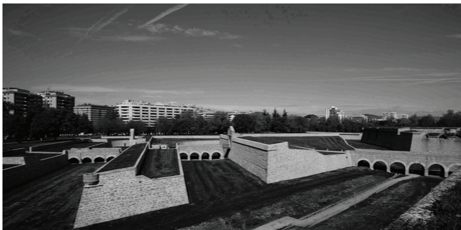
Figure 8. Santa Isabel Ravelin: after the restoration works.
