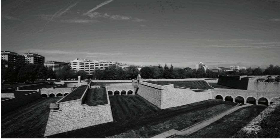
Figure 8. Santa Isabel Ravelin: after the restoration works.
