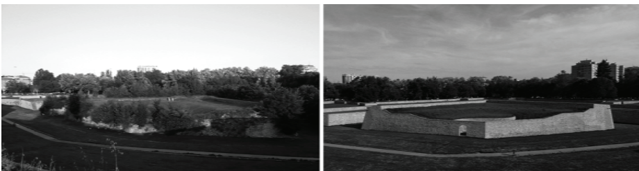
Figure 6. Santa Clara Ravelin: before and after the restoration works.
