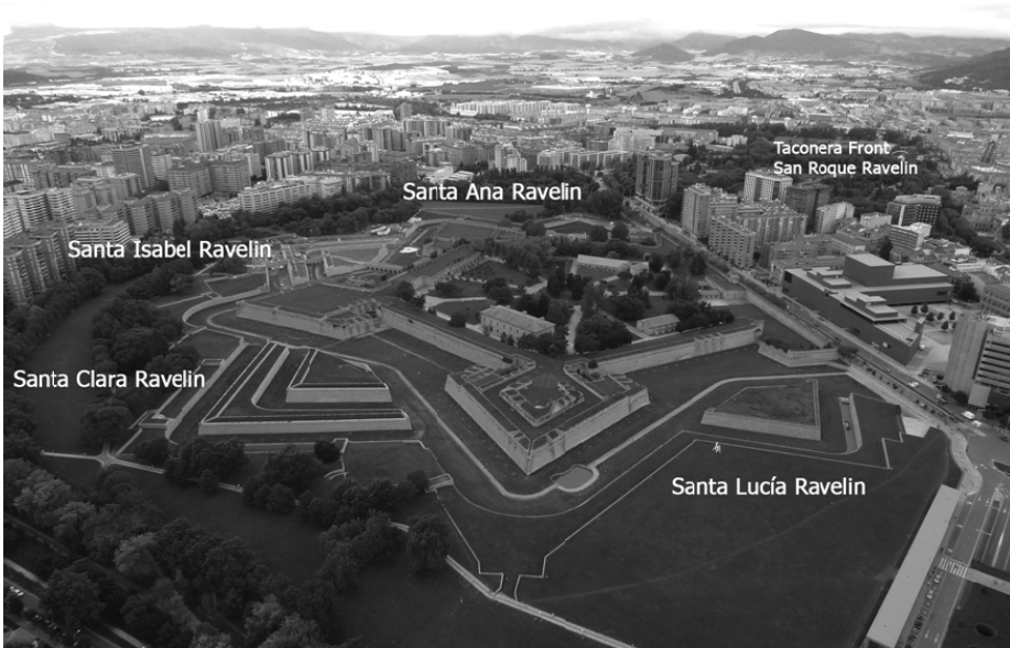
Figure 4. Citadel of Pamplona during the restoration work.
