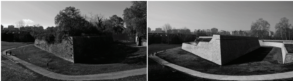
Figure 9. Santa Ana Ravelin: before and after the restoration works.
