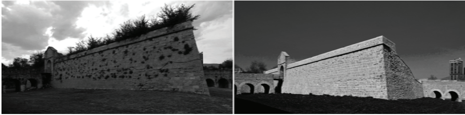
Figure 7. Santa Isabel Ravelin: before and after the restoration works.
