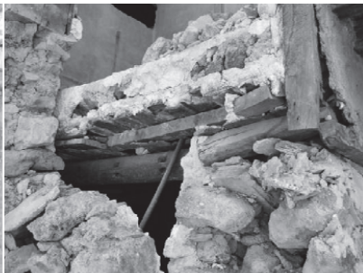
Figures 16 & 17. Floor beams.
