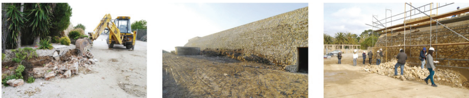
Figure 8. Preliminary work developed out of the walls.
