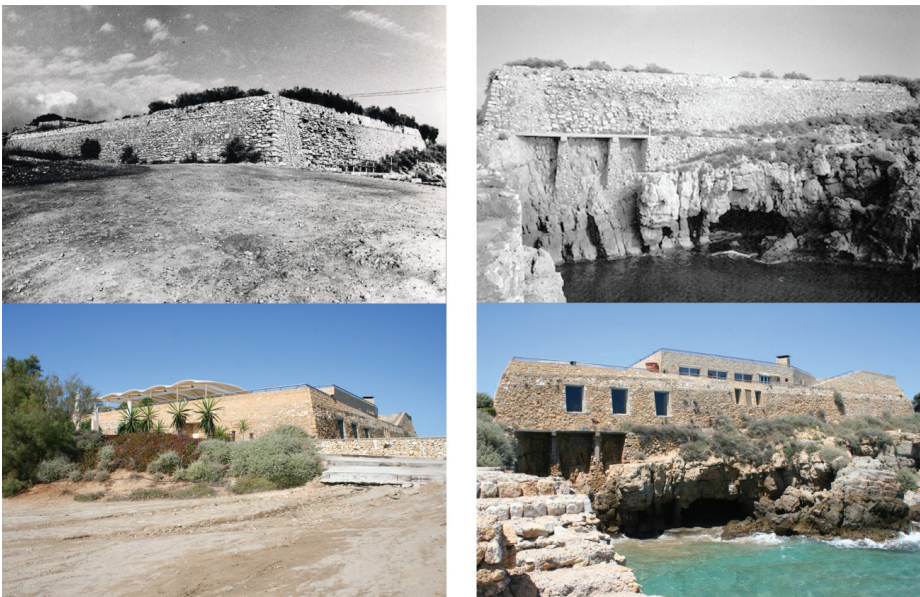
Figure 2. Queen's Fort transformation due to the construction of the restaurant. Comparison between historical images and its appearance in 2007.
