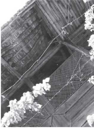
Figure 36. Case02 Timber roof structural elements and wooden fences.
