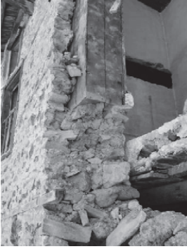
Figures 10 & 11. Masonry and Wooden Frame (Himis) Wall Examples.
