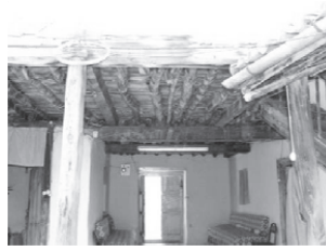
Figure 28. Case01 Floor structure.
