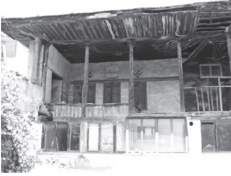
Figure 61. Case09 Courtyard View of the building.
