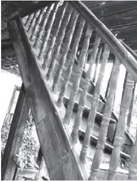
Figure 20. Detail of the Stair steps and the balustrades.
