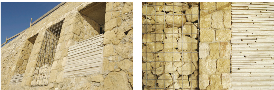
Figure 13. Tests for the outer walled up.
