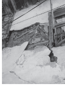
Figures 10 & 11. Masonry and Wooden Frame (Himis) Wall Examples.
