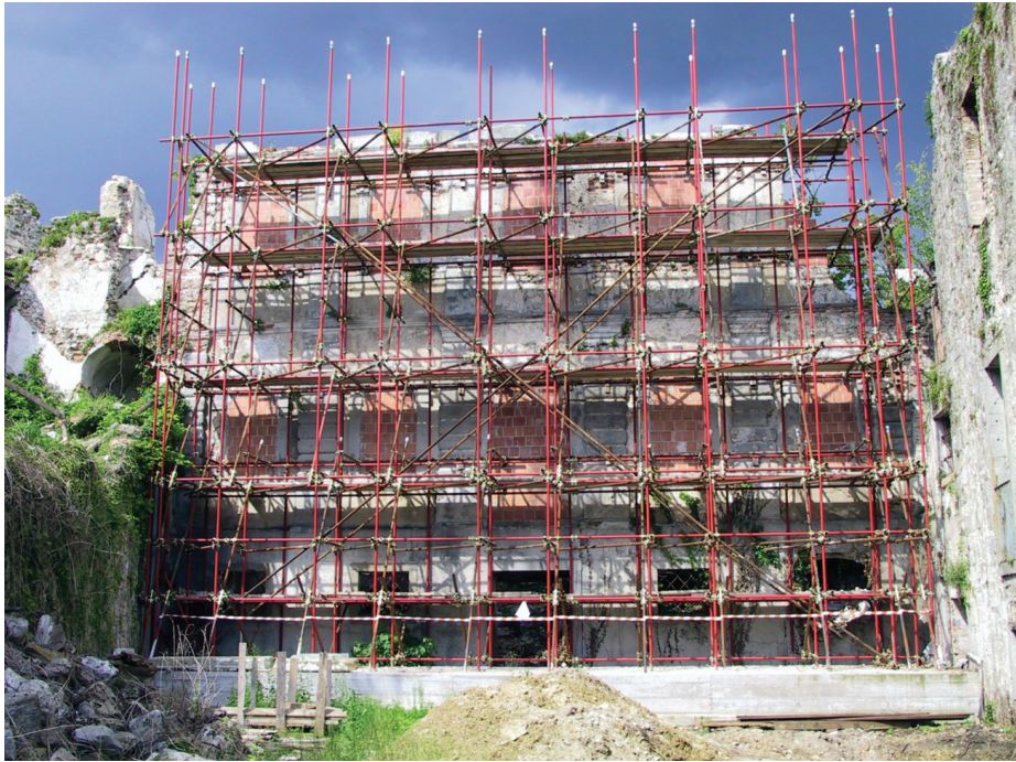
Figure 17. The west front of the East wing, present condition.
