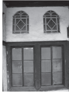
Figure 19. The Sash window and upper windows.
