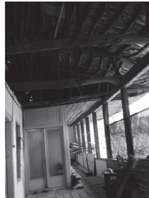
Figure 35. Case02: The external sofa and the roof structure of the building.
