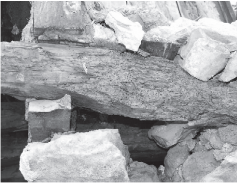
Figure 63. Case09 Case09 The reduced cross-section timber element, causes of insect invasion.
