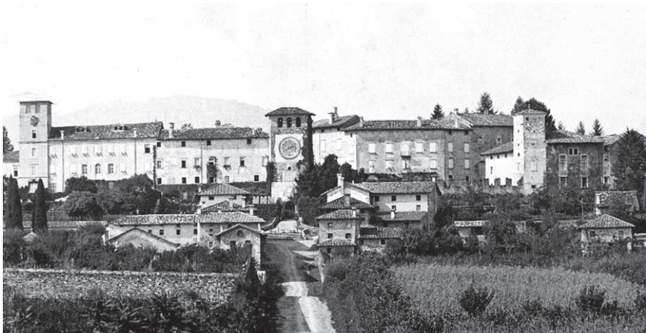
Figure 3. The south front of the castle before the earthquake.
