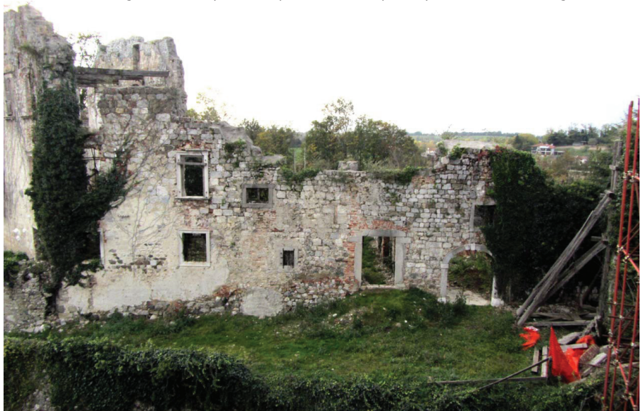
Figure 11. The East front of the Keep, present state.
