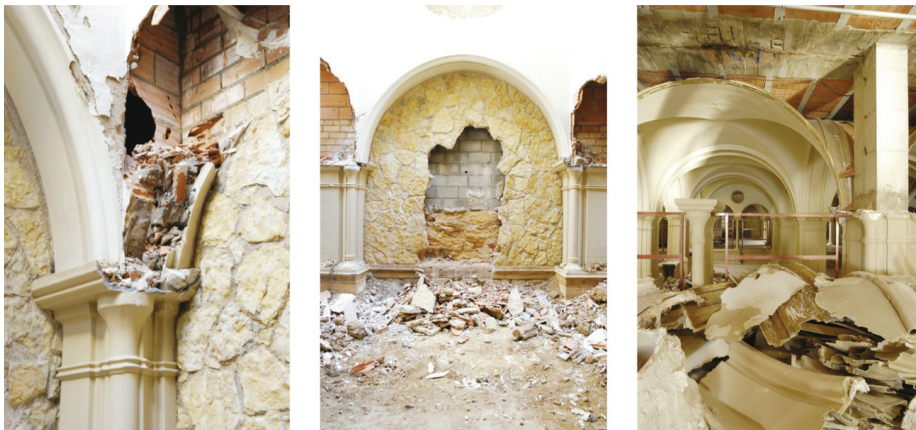
Figure 9. Dismantling decorative veneers.
