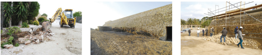
Figure 8. Preliminary work developed out of the walls.
