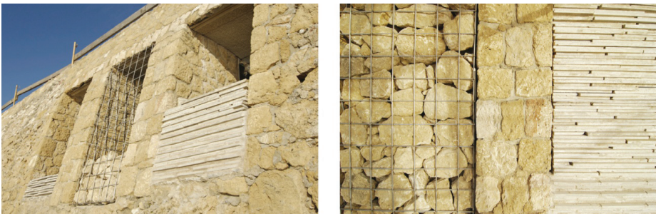
Figure 13. Tests for the outer walled up.
