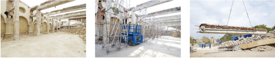
Figure 11. Dismantling and removing the large beams from the east hall.
