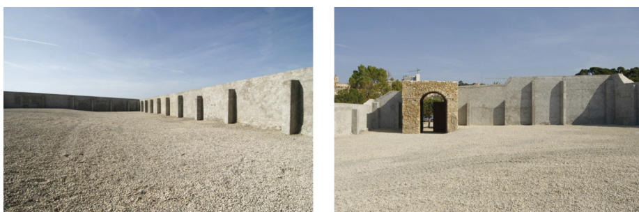
Figure 14. Interior of the Fort after the demolition and consolidation works.
