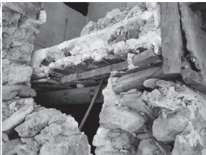
Figures 16 & 17. Floor beams.
