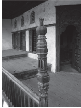
Figure 21. Capital of the wooden balustrade.
