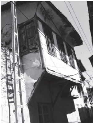
Figure 34. Case 02: The entrance façade of the building.
