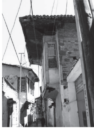
Figure 37. Case02 The building and its surrounding.
