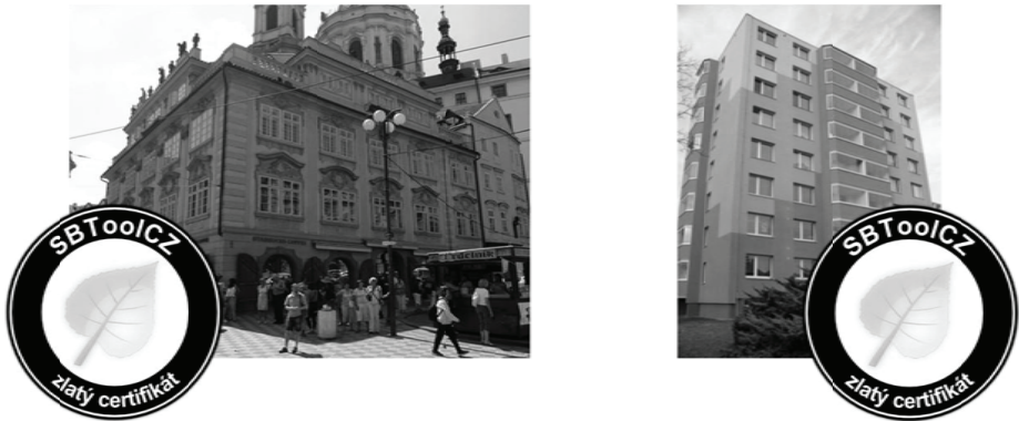
Figure 3. Listed building after BAT renovation and renovated building without historical protection with parameters as a new building.
