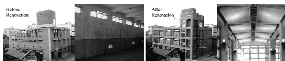
Figure 1. Wine storage warehouse before and after renovation.
