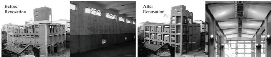
Figure 1. Wine storage warehouse before and after renovation.
