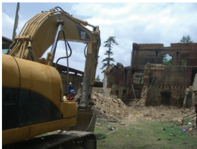
Figure 10. Overview of pull-down test.
