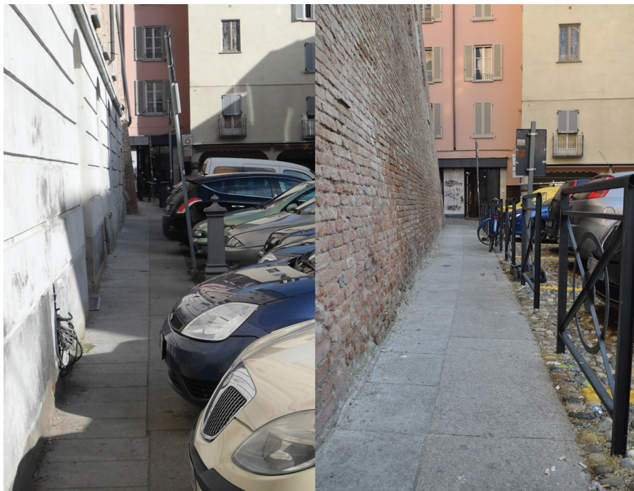
Figure 6. Piazza Cavagneria: how it was before and how it is now; the Municipality realized the idea we designed even if the elements to preserve the path are made by iron (in our project they were thought in corten) and their geometry is different (they are 1.10 m height while the corten panels in the project were 0.45 m).
