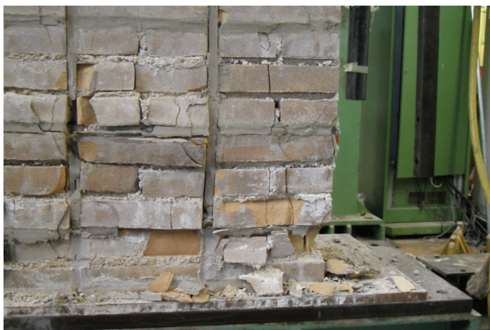
Figure 9. Cracks appeared on bricks of reinforced samples subjected to vertical compression test.
