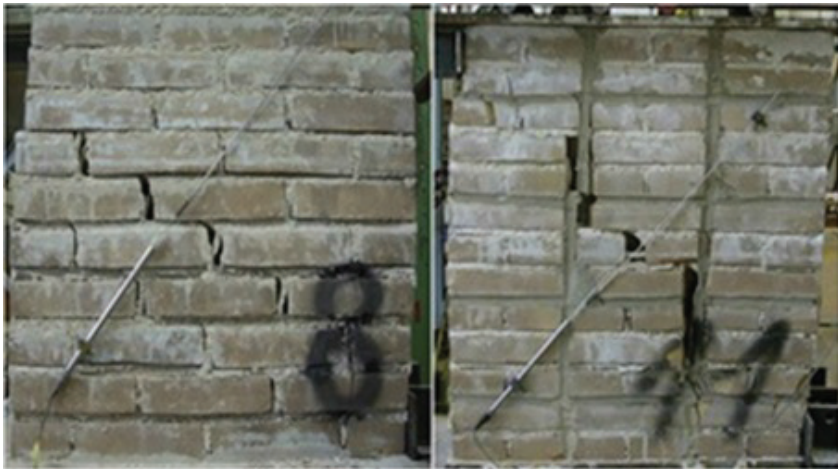
Figure 11. Three-leaf masonry samples after shear-compression test: on the left the unreinforced ones ("NC") and, on the right, the ones strengthened through BF arranged both horizontal and vertical bed mortar joints ("RR").
