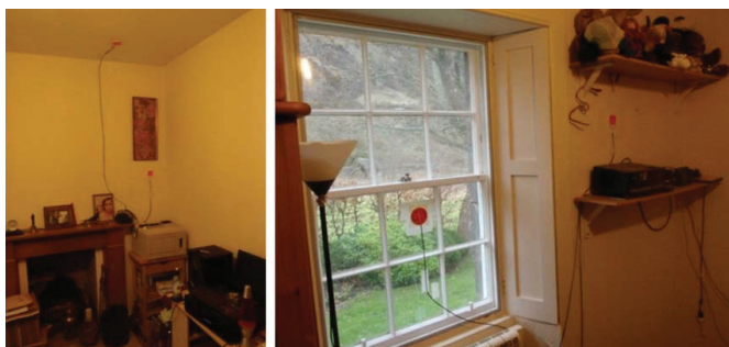
Figure 4. Heat flow mats on north east wall & window.
